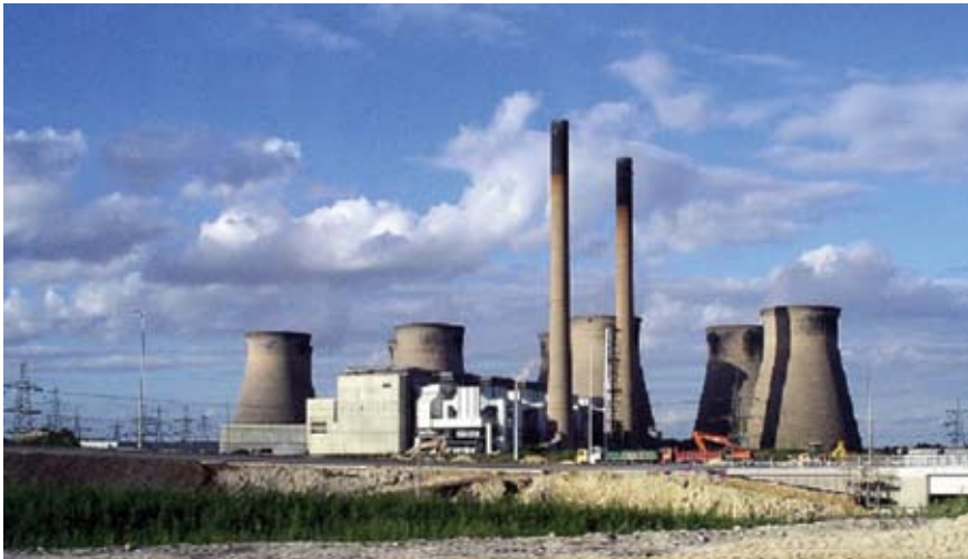
UK Utility 4x500 MW e 4x1350MW th Coal with 2x6x25MW th Wood Pellets Bioswirl
